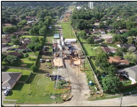
36" corridor project in the Houston area. Pictured is a HDD operation.
