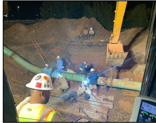
Tony's Crew tying in a valve setting. Pictured is Swamper -Eric Tello, Welders - Sherman Kitchens, Andy Neel, Brian Neel. WH - Arnold Lopez, Jonathon Svoboda, Cameron Neel, Miguel Rivera. Foreman Americo Lucero and Julio Alanis oversee the work. Picture by Kelly Ellis - Operator.
