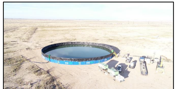
Lake Tank used by crew in Artesia, NM to provide the water for hydro-testing.
