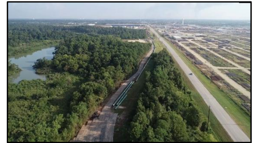
36" pipe strung and welded on project in the Houston area.
