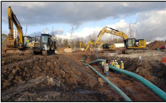
Crew's lowering in pipe to prepare for a tie in.
