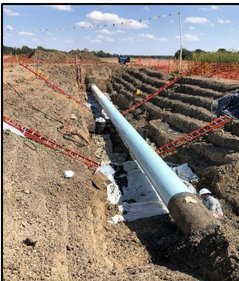
Cut out and recoat project.
