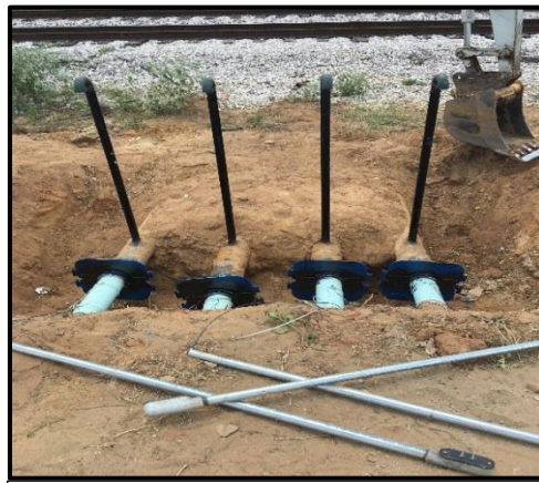
Installation of four end seals.
