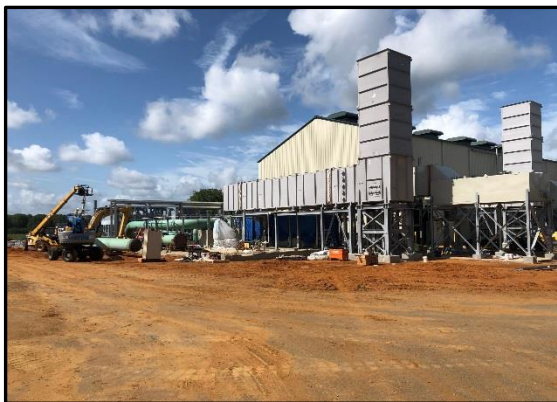
Set Intake and Exhaust Structural Steel and Ducts for the Mars 100 Turbine Package.
