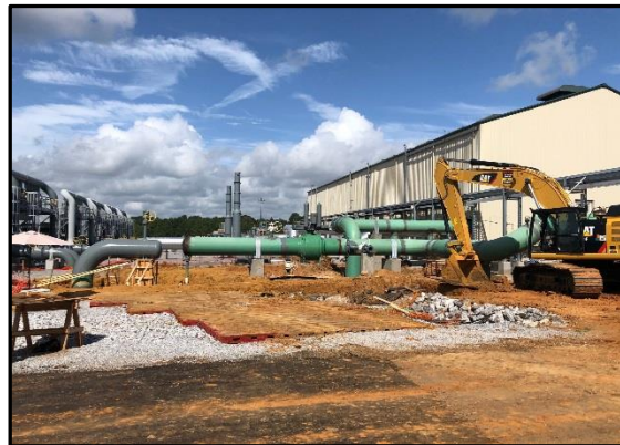
36" Suction and Discharge Pipe in Preparation of the 8 Hour Hydrotest.
