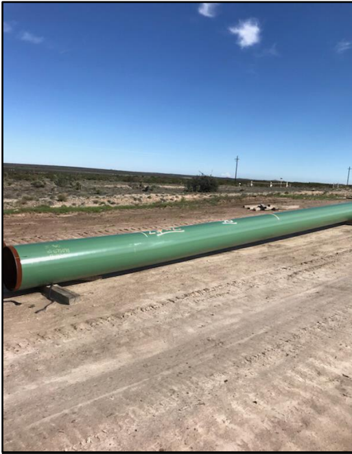
Pipe on the 24" project.
