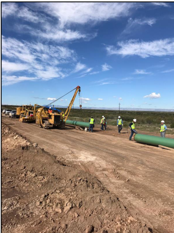
JJ Harpole's front end crew on the 24" job.
