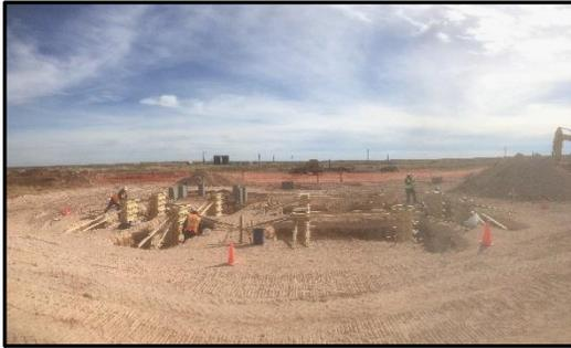
Rojo Toro Meter Station. Concrete crew building piers for the Meter Station.
