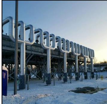
Gas cooler in Owensville. Completed picture of Gas cooler piping in Owensville Compressor Station.
