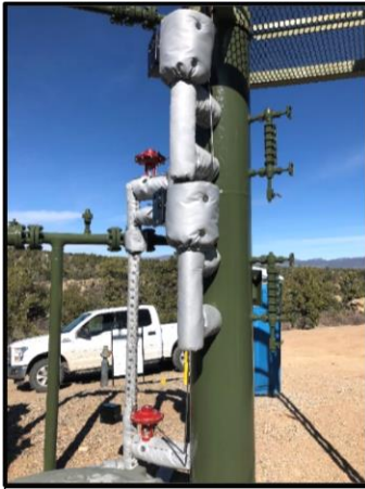
Insulation for FMOA project.
